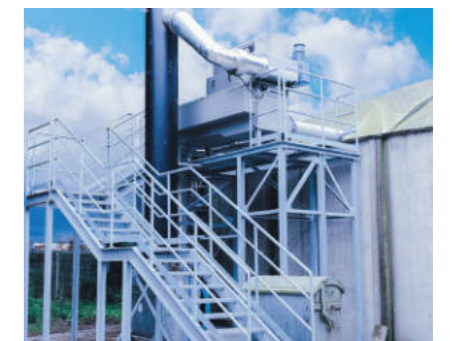
Steelwork structures and platforms
