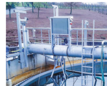
Scraper – as round and long basin scraper for removing of sludge, grit and floating materials
